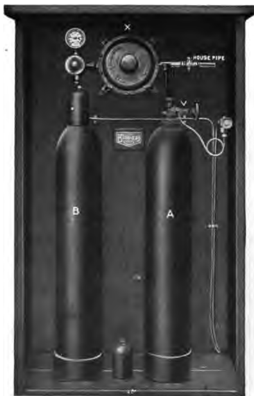
FIG. 75.—Blaugas cylinders. Pipe at right leads to underground expansion tank.
